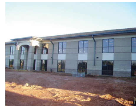
Completed in 2009, a new 63,000 sq. ft. facility positioned The Mill for continued growth.
